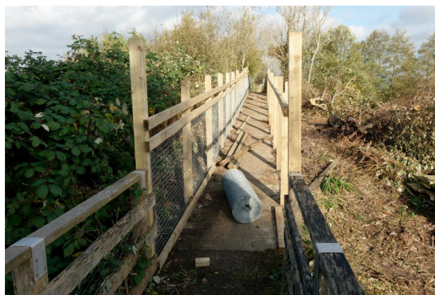
The new footpath fencing – in progress (photograph by Geoff Carefoot).
