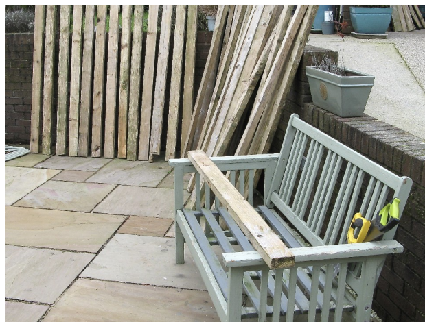
Recycling timber, from the old footpath fence, for the construction of the nesting bank (photograph by Geoff Carefoot).
