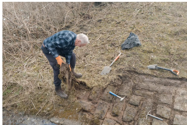
Exposing stonework on one of the spillways.
