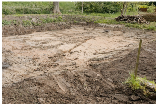
The newly dug pond.
