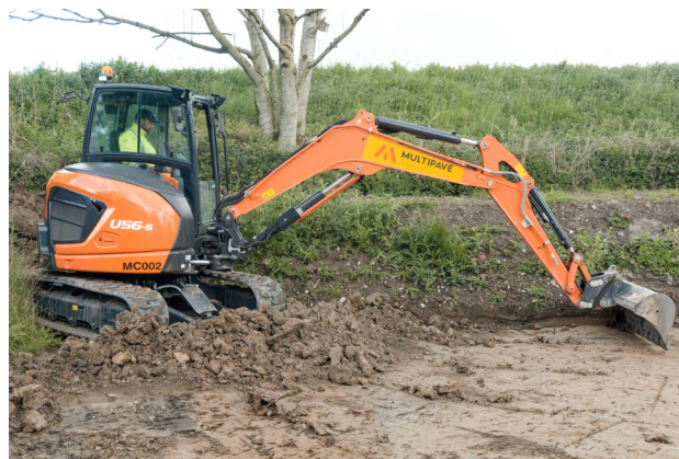
The Multipave team at work on the new pond.
